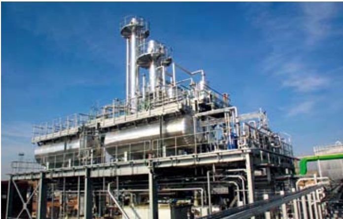
Caparroso biodiesel plant in Spain. Photo: Acciona
